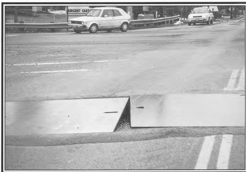
It's a good idea to stay away from the edges of steel construction plates.
